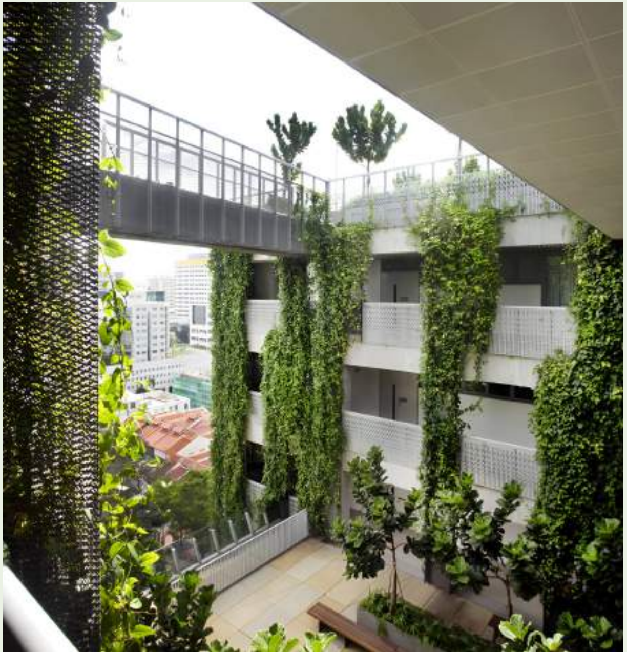
The Singapore School of the Arts by WOHA, Photo by Patrick Bingham Hall
