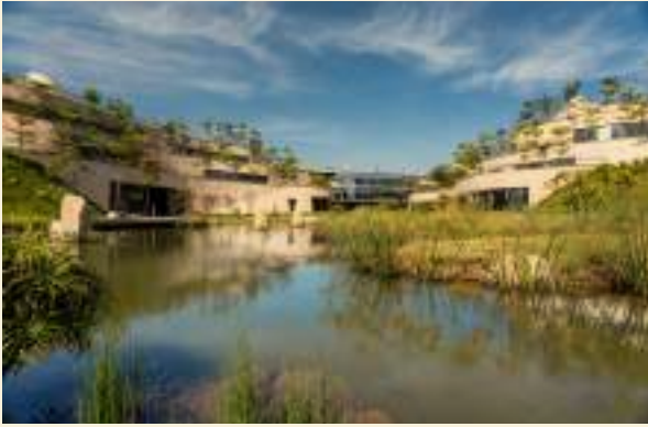
Titan Integrity Campus
