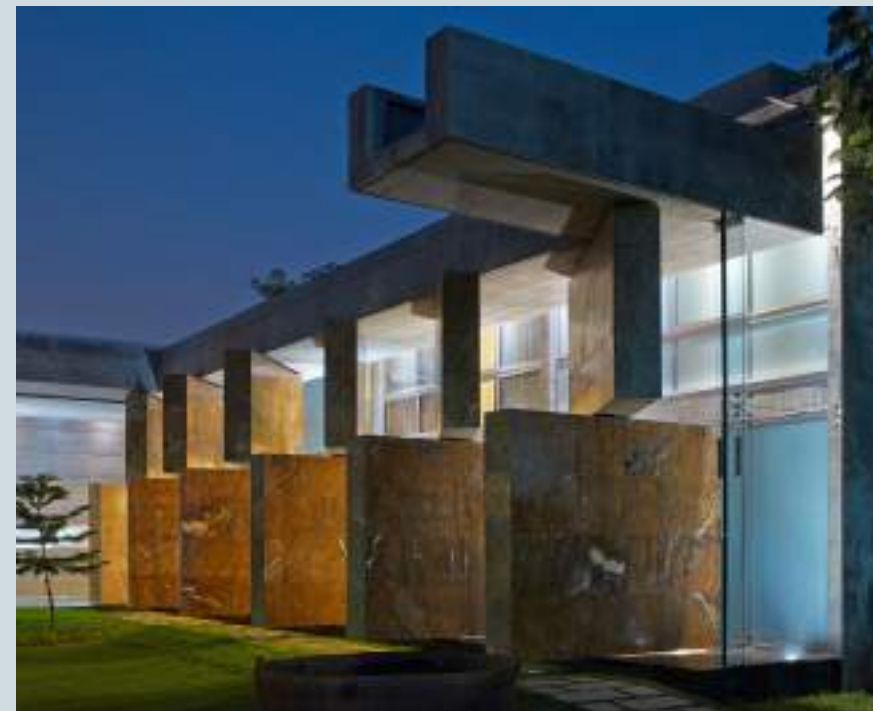
Large stone walls can be easily pivoted to allow the passage of light, air, people and more. Photo Credit: Edmund Sumner
