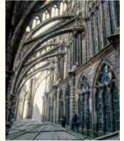
Flying Buttresses of Amiens Cathedral
