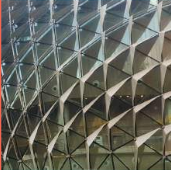
Openings at the Esplanade Theatre, Singapore, designed by DP Architects and Michael Wilford. The theatre's distinctive glass domes have an elaborate external shading system. They consist of triangular metallic louvres that adjust according to the sun's movement, mimicking the spiky exterior of a durian fruit.
