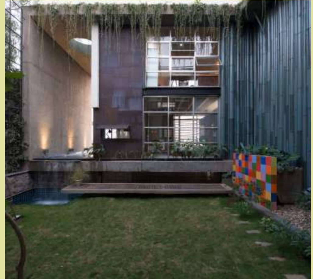
The courtyard from inside and outside. Resting over the rainwater harvesting tank that is scooped from the bedrock.
