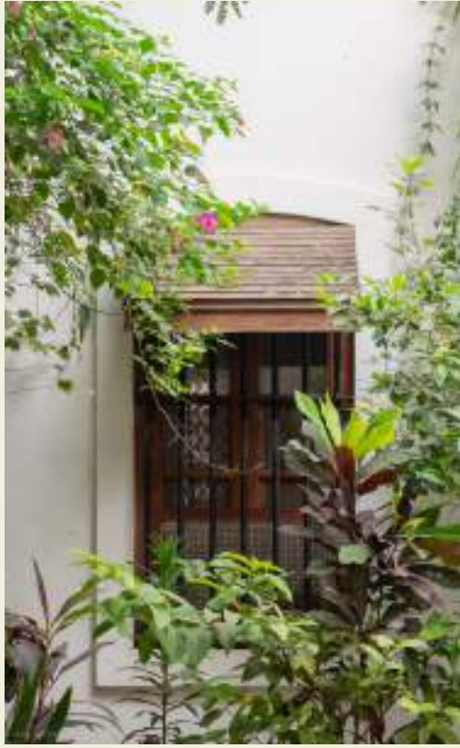
In modern-day Pondicherry, French colonial styles blend with traditional Indian materials such as terracotta tiles and wooden screens, resulting in openings that offer privacy, ventilation, & light.
