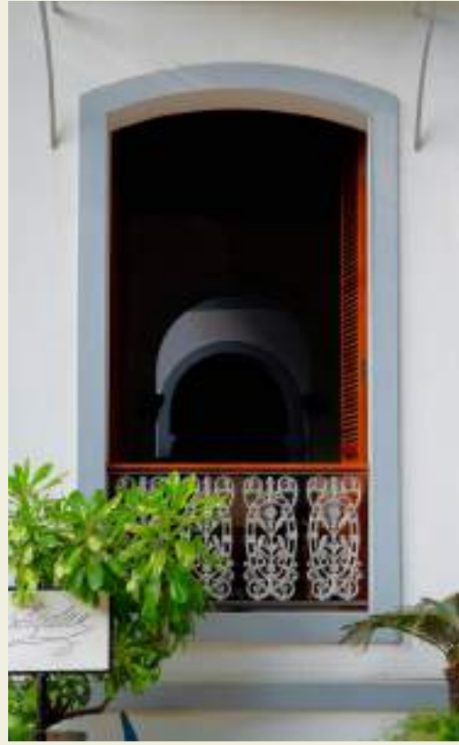
An arched window with wooden louvred shutters and a beautiful, ornamental metal railing. The opening gives you a hint of what lies inside.
