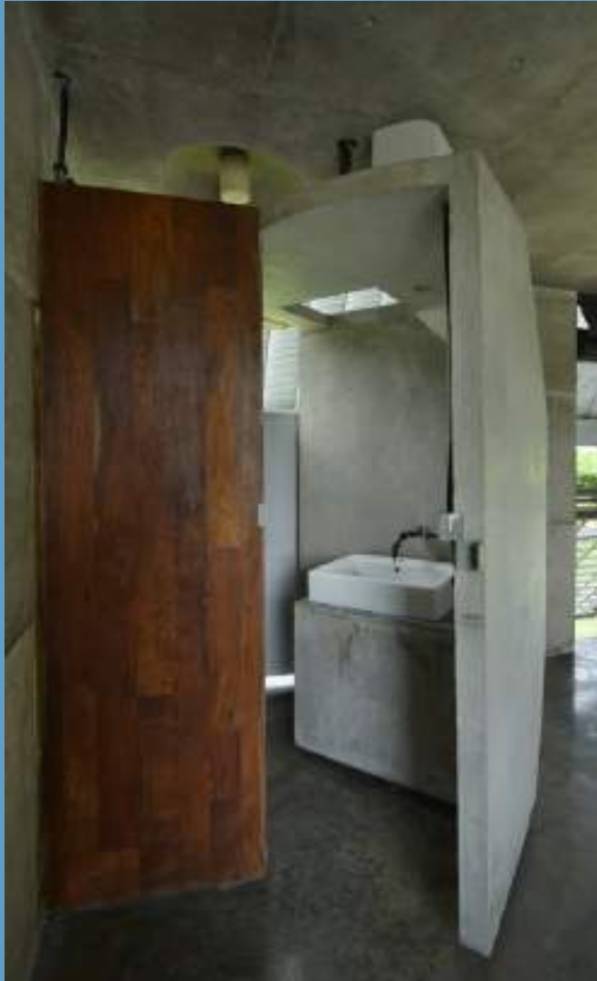
What looks like the door is stationary, surprise!!! The entire set-up of the wall and water closet moves! Photo credit: Matharoo Associates
