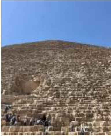
Entrance vault of the Great Pyramid
