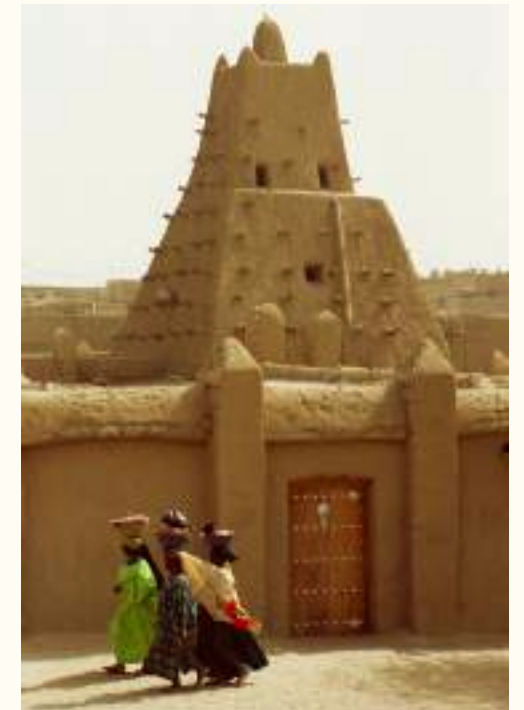
Small openings in the adobe walls of Sahelian Architecture
