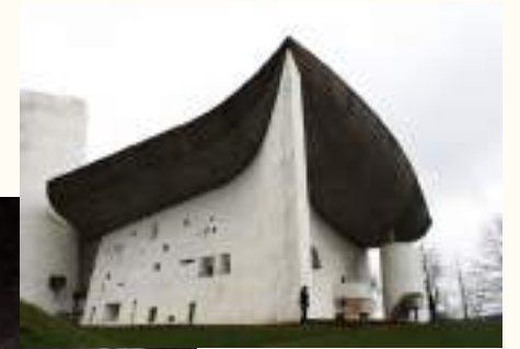
Facade with penetrations
