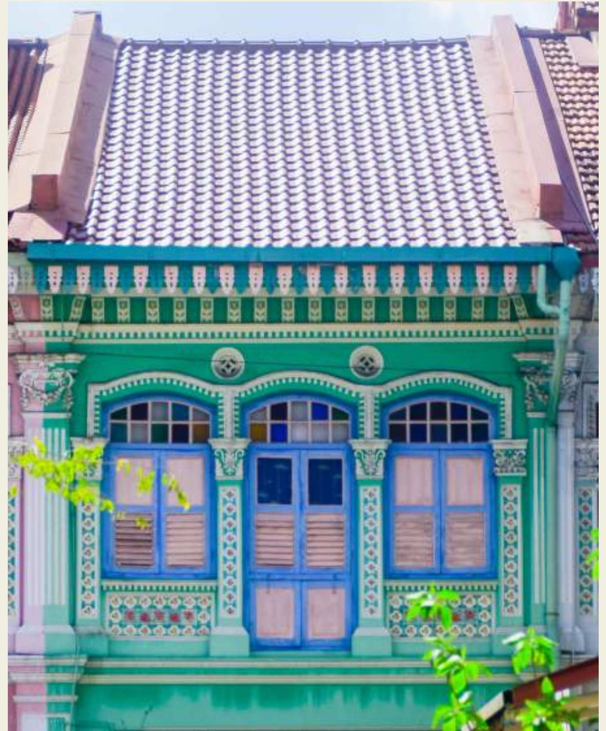
Shophouses of Singapore, with their colourful wooden doors and windows.
