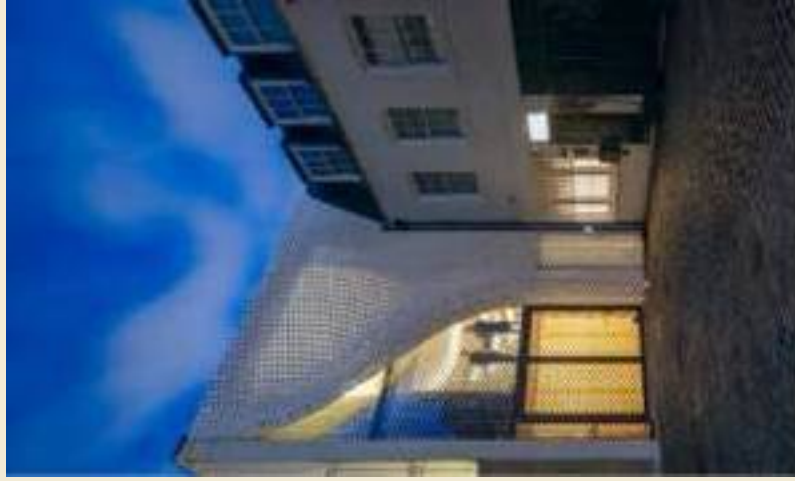
The facade reveals a dynamic interplay of open and closed spaces through a carefully patterned brick course. This self-supported wall, anchored to the glazing plane at critical points, exemplifies our commitment to pioneering future architectural language. Photo by Luke Hayes
