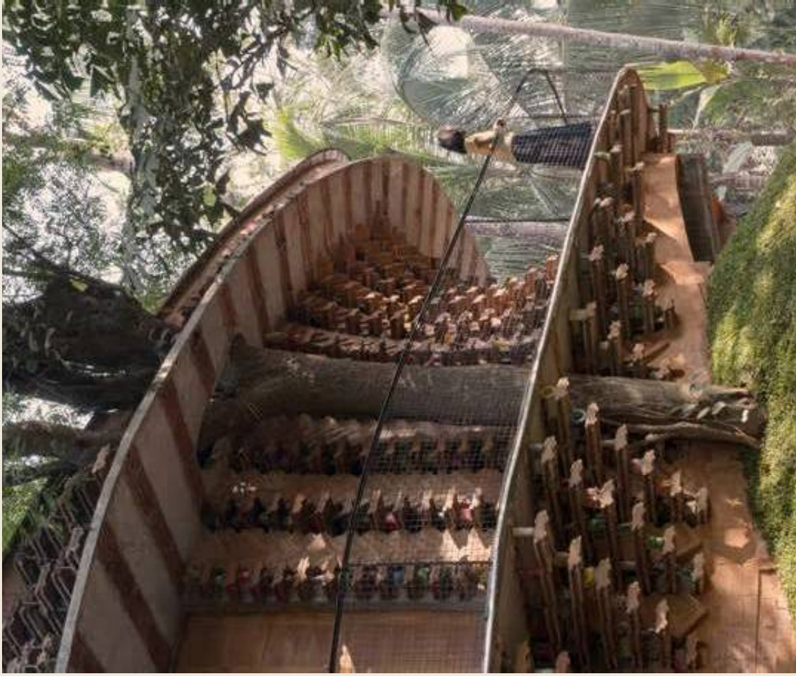
Toj Storey Kerala | 2021 Toj waste integrated into wall construction.
