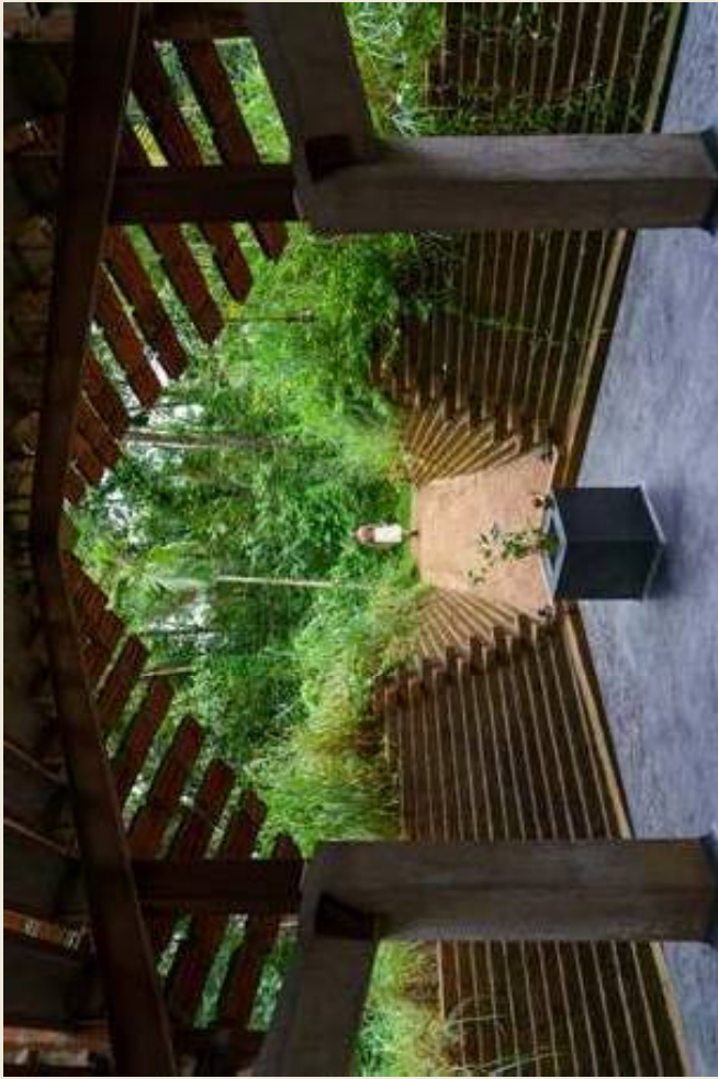
Chirath, Kerala | 2018 Remnants of pit and scrap materials seamlessly integrate into the walls of this project, defining spaces & facilitating ventilation and enhancing natural lighting.
