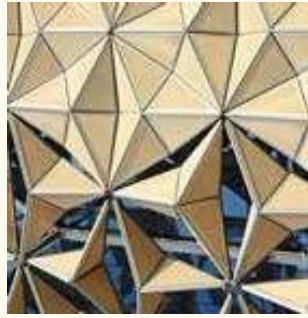
The world's largest computerised facade / kinetic on the Al Bahr towers in Abu Dhabi.
