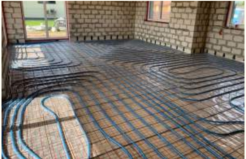
Underfloor heating installation
