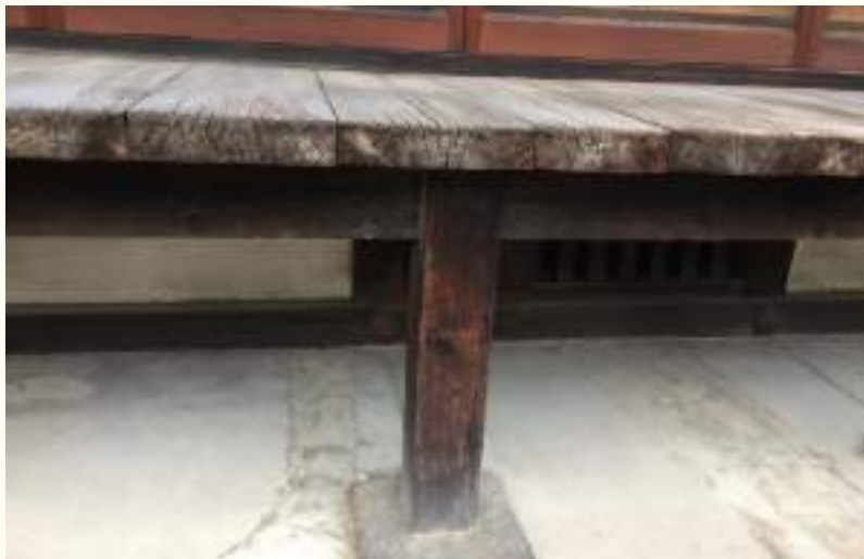
Bracket from underneath that supports the floorboards
