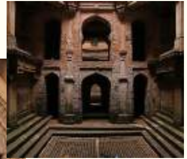
View of the stepwell stairs
