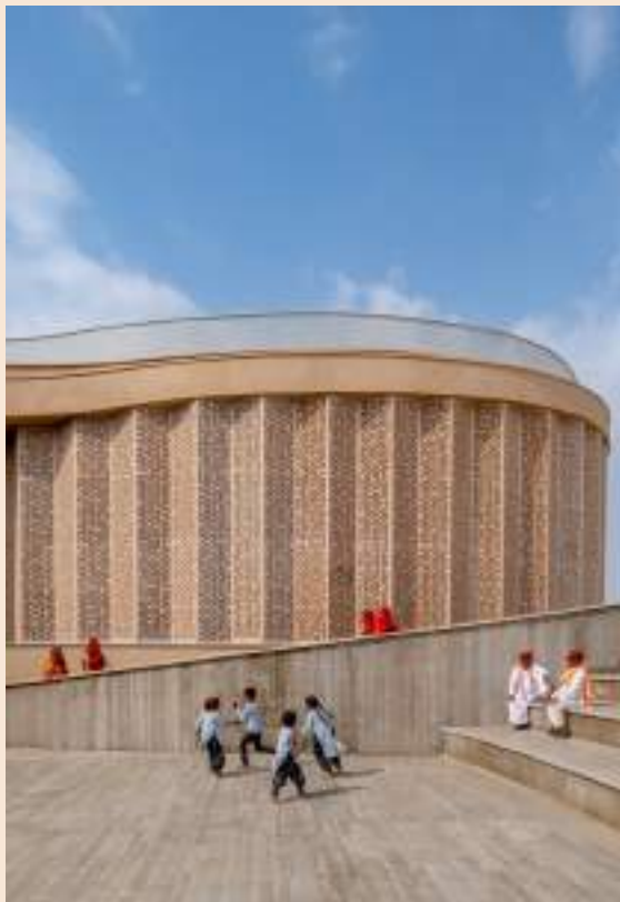
One floor, many possibilities, what begins as a foundation multiplies into gardens, amphitheatres, and sheltered havens, turning ground into a launchpad for life.
