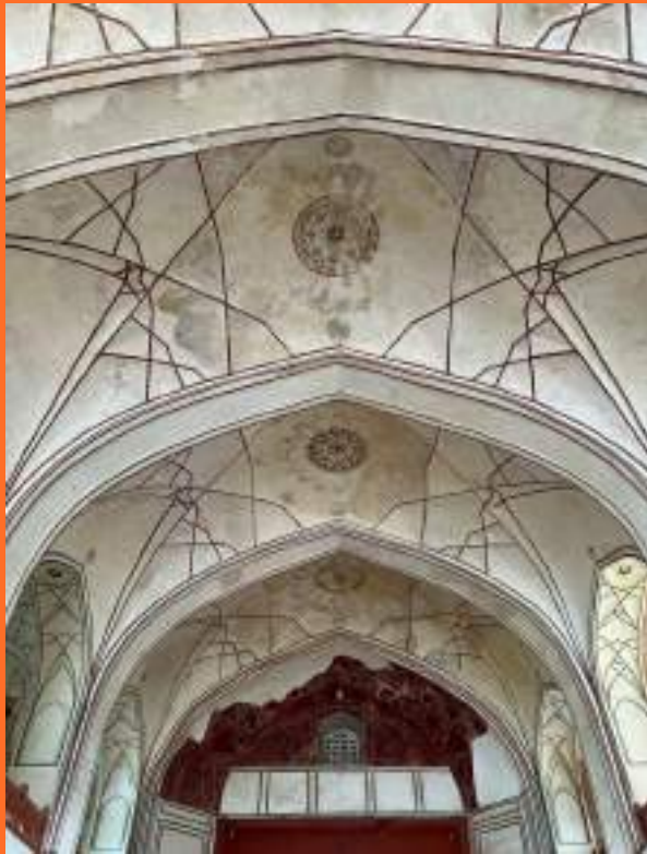
Decorated ceiling of a domed roof with radiating ribs, Red Fort in Delhi. Photo by Nard Get
