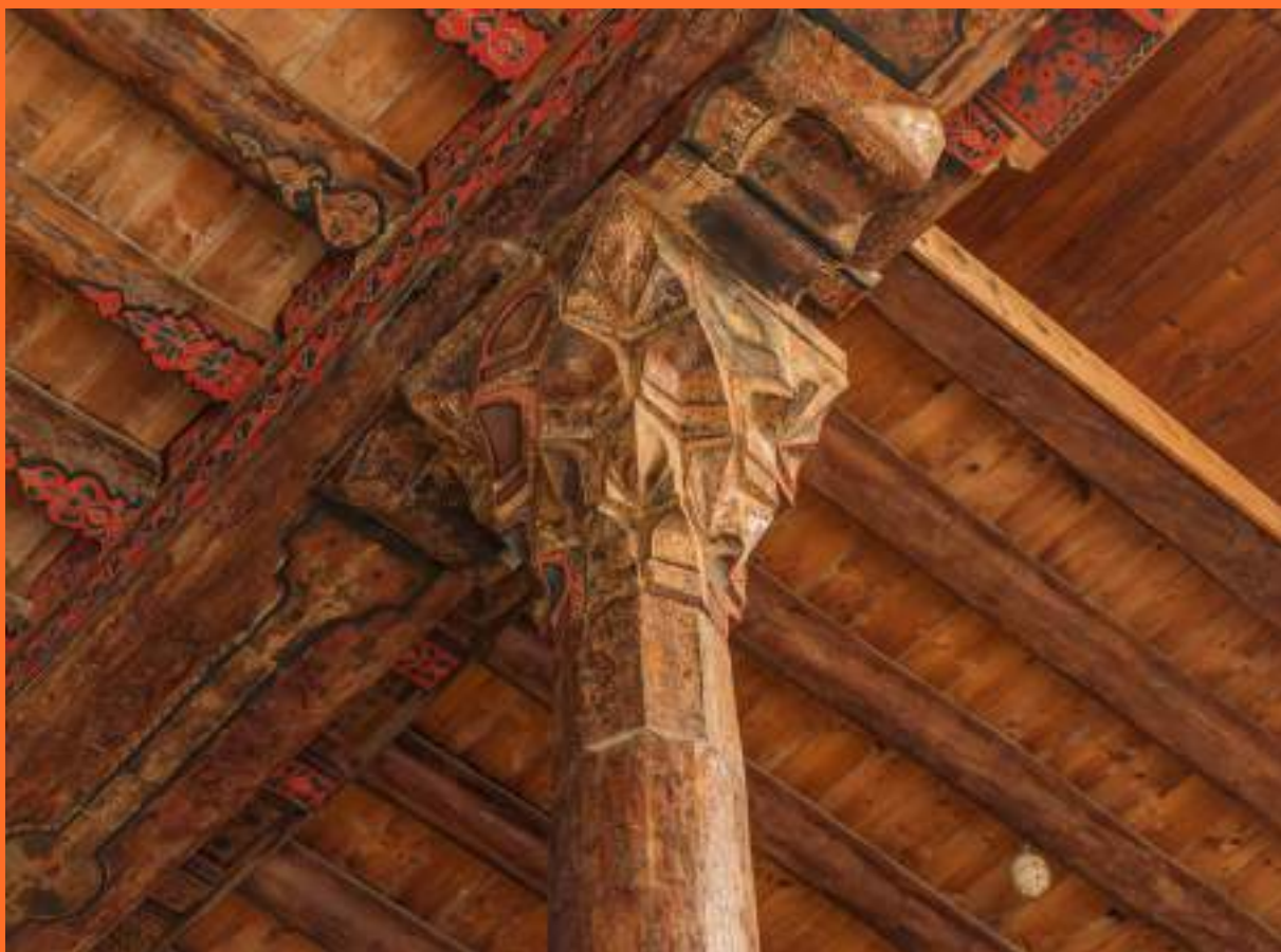
Columns, beams, and purlins frame the ceiling of an intermediate floor in Eşrefoğlu Mosque, Turkey. Photo by Mahmut
