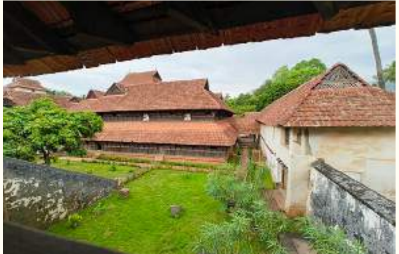
Vernacular terracotta roof of Padmanabhapuram Palace
