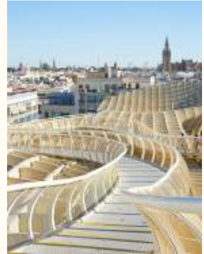
The walkway atop the parasol
