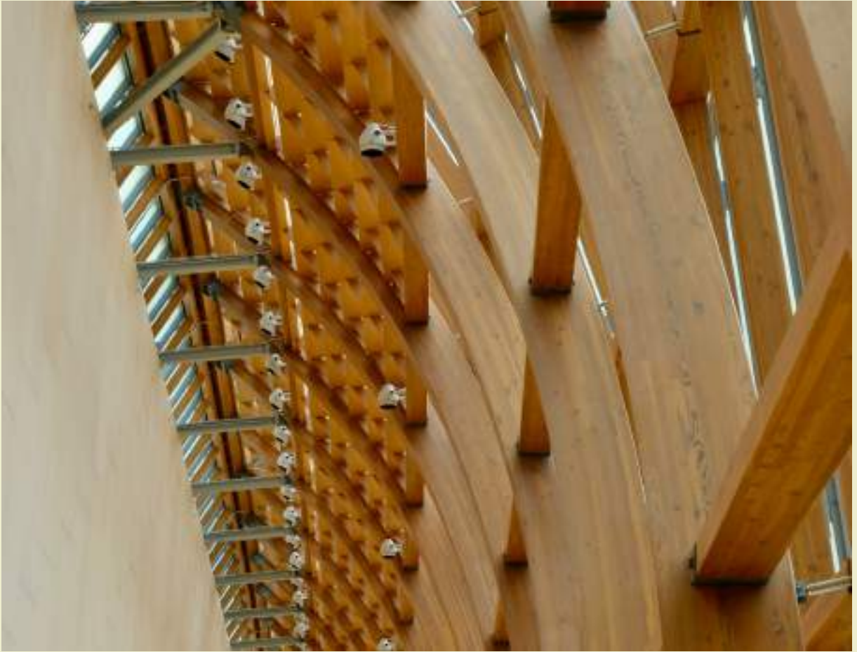
Ceiling of a sloping roof with timber trusses at Art Gallery of Ontario, Canada. Photo by Anil Baki Durmus
