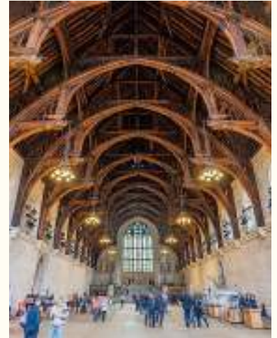
Hammer-beam roof of Westminster Hall
