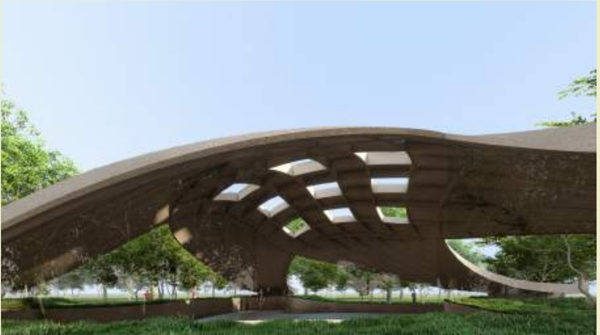
View from the grid shell roof of the Experience Centre at Sakleshpur. ©Play Architecture
