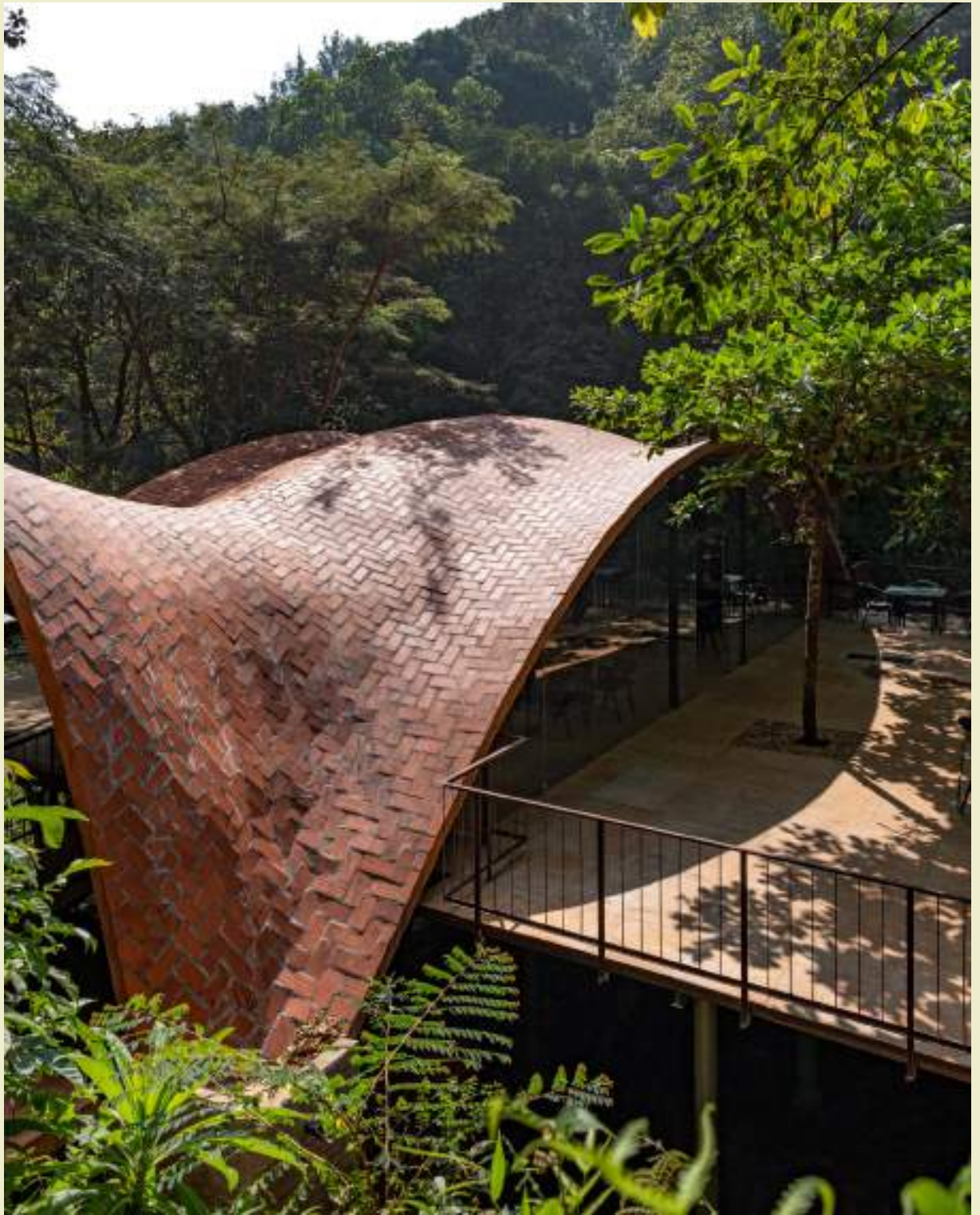
Aerial view of the vaulted dining space at Devadhare. © Bharath Ramamrutham, GRAF Media.
