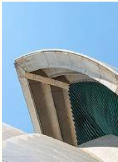
View of one concrete shell
