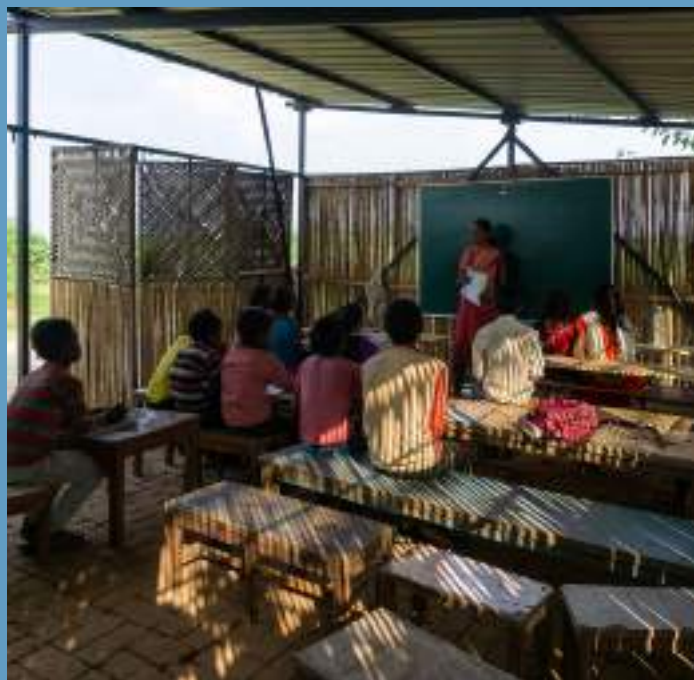
Our collaboration with the farmers began in 2016-17, designing and rebuilding a school using local materials for their children after it was demolished by the planning authorities.
